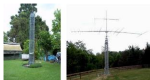
Figure 350-65: Amateur Radio Antenna Support Structure (Crank-Up Tower)
